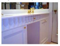
The client liked it so much he decided not to have the plaster fluted moulding in the room. Instead, he wanted me to make sections of matching wood moulding! I mitered them on the bottom to make a double scallop. We used adjustable sized corner blocks in the room so full-size flutes could be used throughout.
